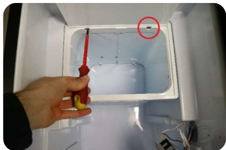
1) Unscrew the evaporator (2 screws)
